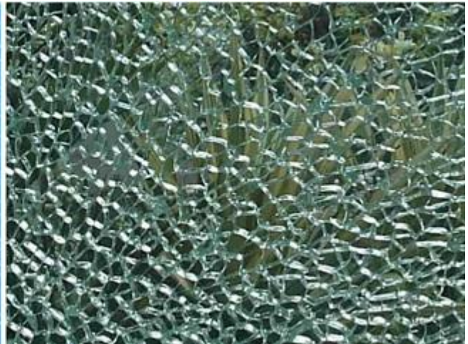
Tempered laminated glass broken
