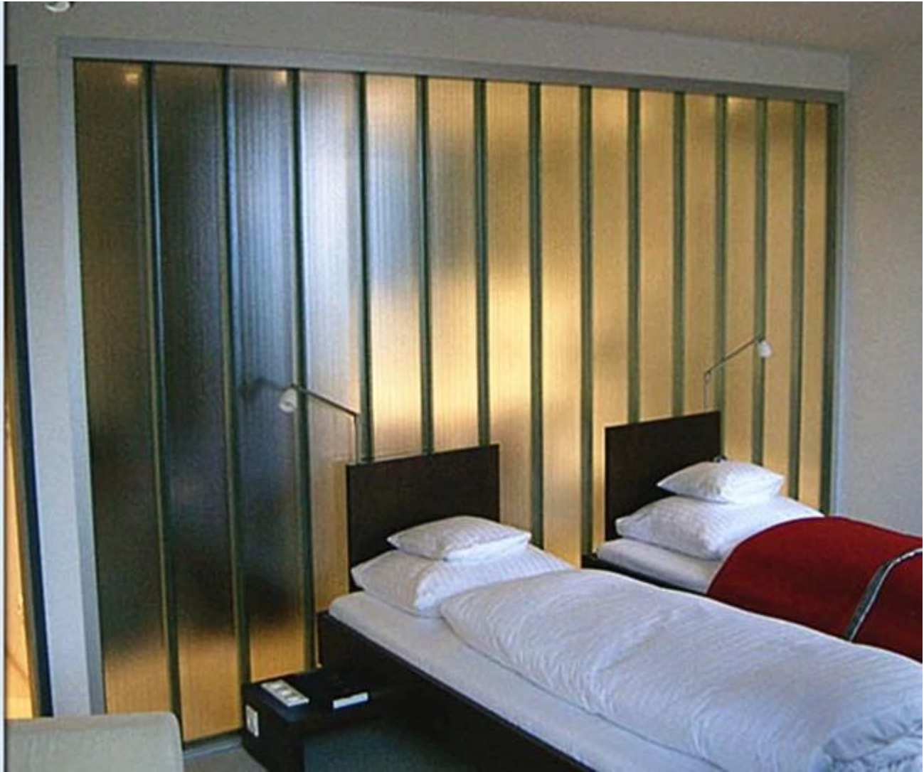
7mm U channel glass curtain wall:
