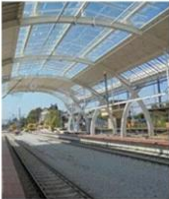
Gliwice Metro Station
